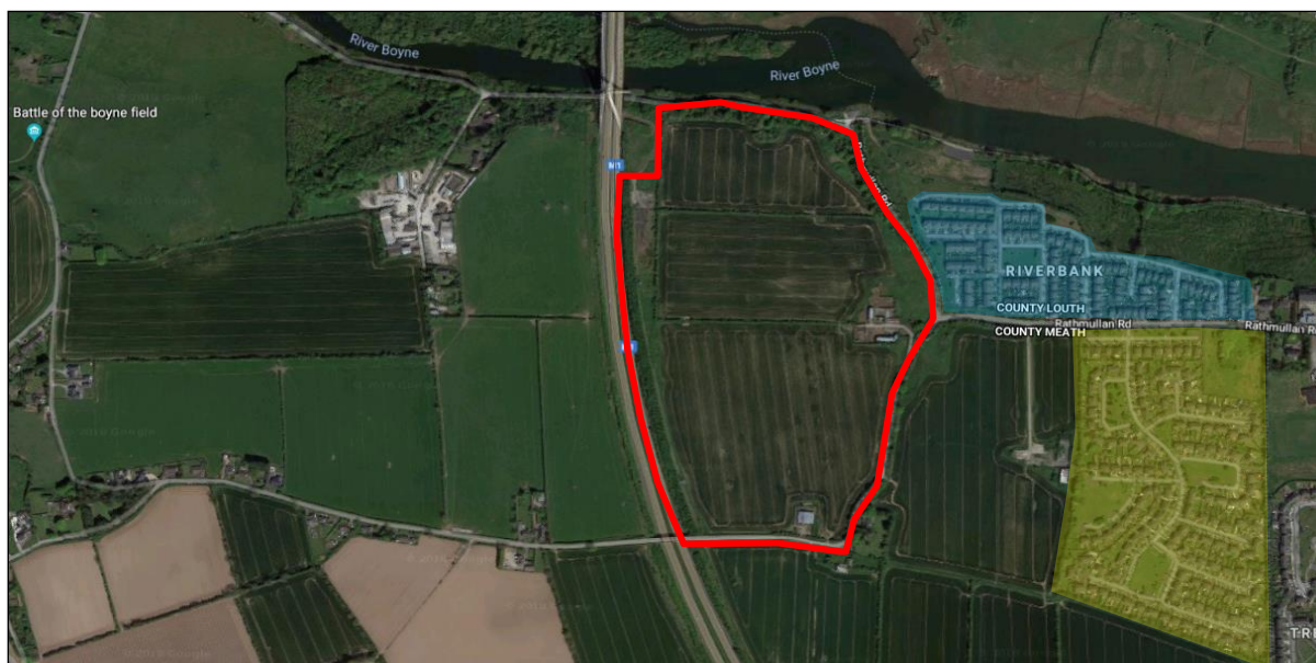
Figure 1.0 Aerial view of subject site (red outline) in the context of the receiving environment with existing housing developments 'Riverbank' and 'Highlands' shown in blue and yellow.
